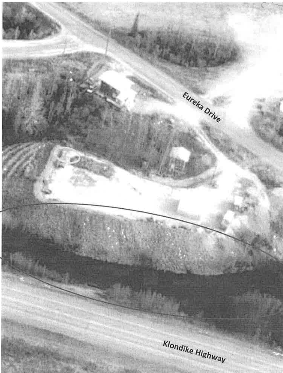
Figure 3: Constraints rendering sections of this lot undevelopable. The red circle shows the steep slope and tailing pond next to the Klondike Highway. The yellow circle shows the approximate location of the septic tank.
