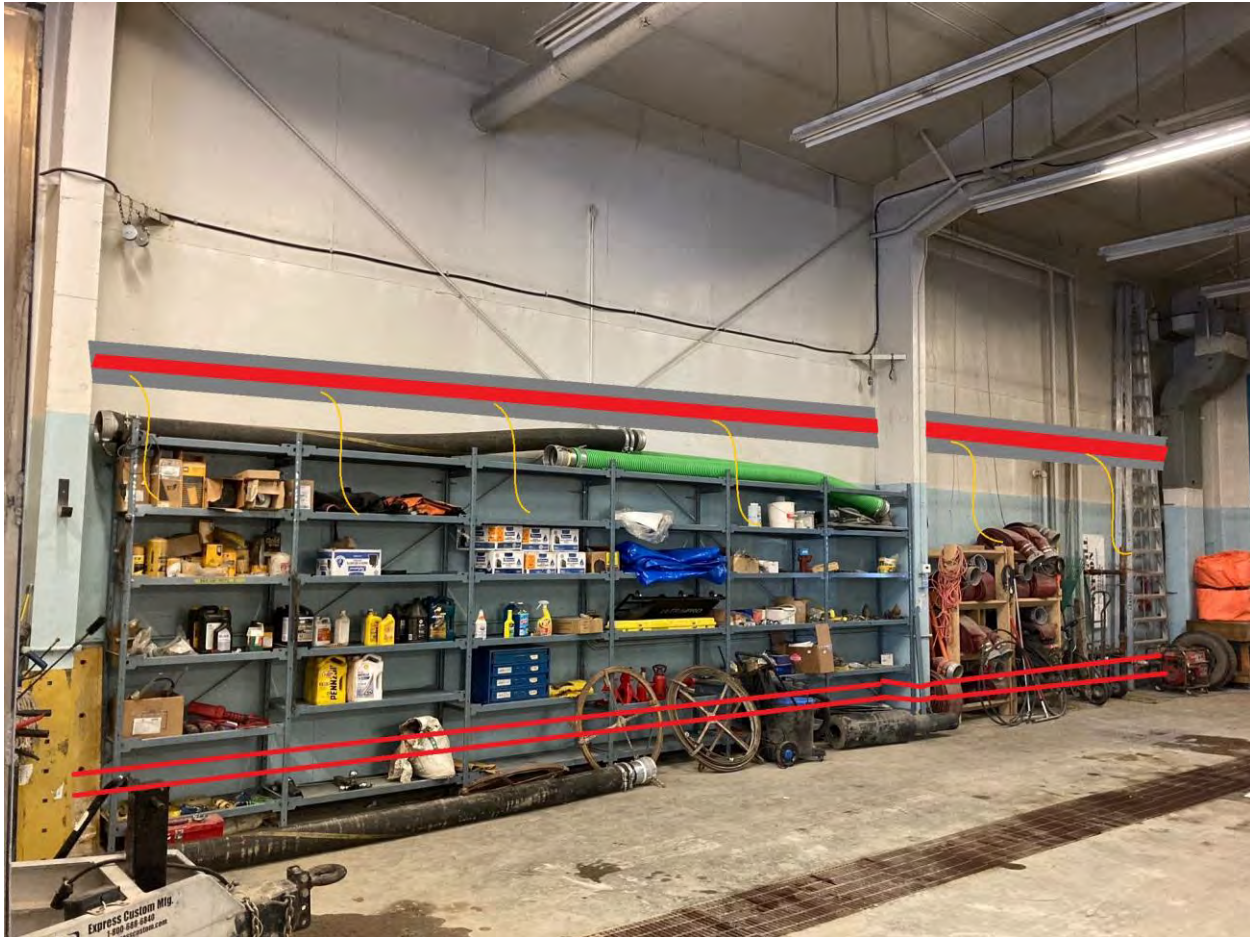
Figure : Radiant heating lines near ground level behind the shelving units are shown in red.
