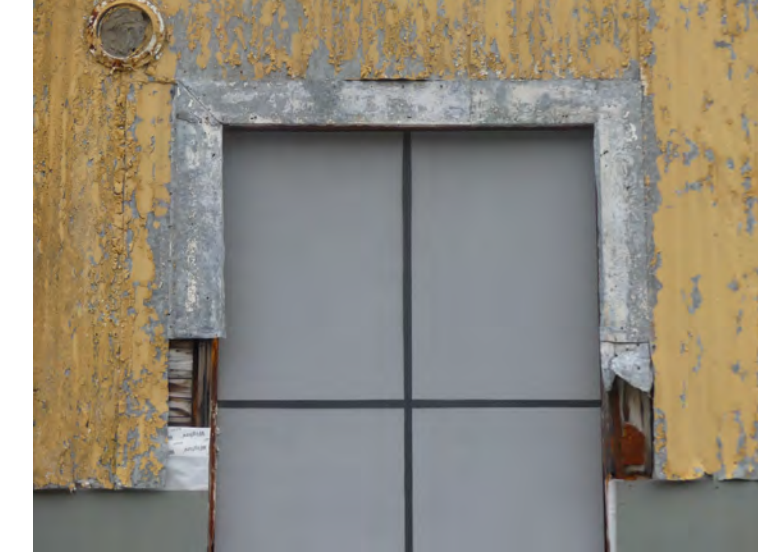
41. window frame, main floor, repair would be straightforward with the metal frame replaced, the chimney thimble would remain
