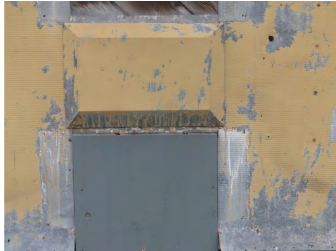
10. Typical small quoin, the surface texture and nailing pattern show clearly. A separate piece of metal is slipped in behind to assist in shedding water
