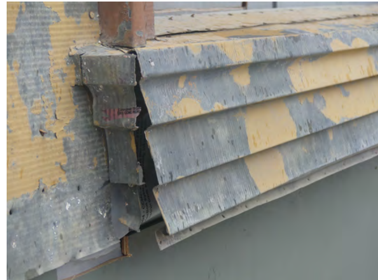
21. the lower windows sills are generally damaged from when the building was raised. Repair or replacement of the sills will require careful disassembly of the adjacent metal siding. Some sills may be repairable in place and resoldered.
