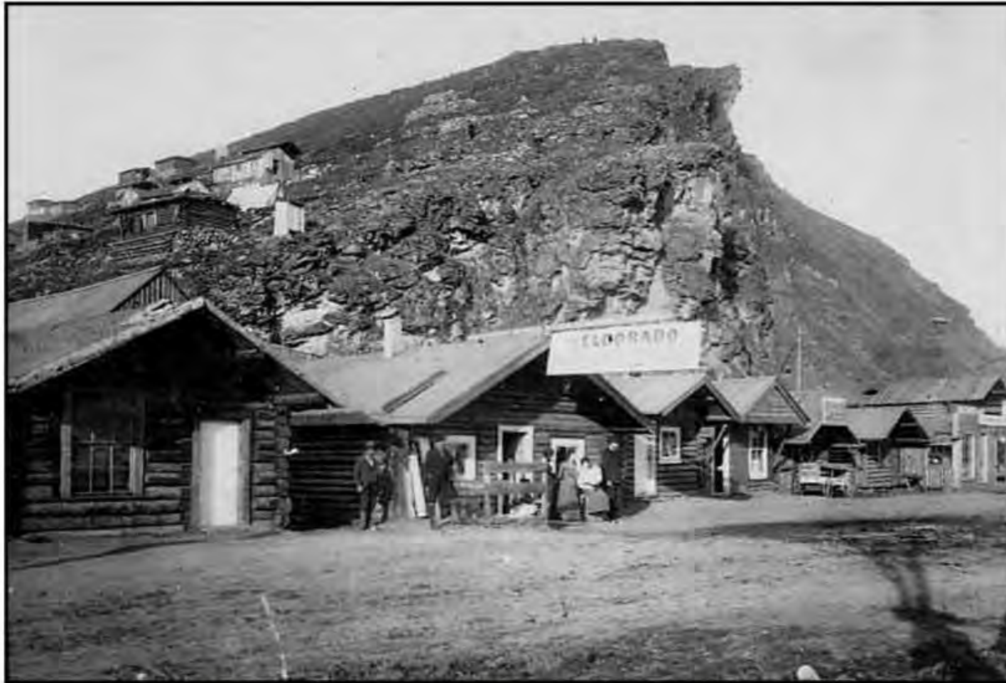
1984.50.23 - Photograph of "The Eldorado Bottling Works." "Under Crocus Bluff (P. Butterworth)." Front Street at Crocus Bluff with small log cabins built along street and up the hill behind. A group of unidentified people is posed at the front of the Eldorado Bottling Works. "Peerless Laundry" and a "Lunch Room" are also advertised along the street. In front of the Peerless Laundry the cart reads "Shore Acres Standard Theatre." Circa 1897-1910. Dawson City Museum and Historical Society, 1984.50.23, The Cribb's Drugstore Fonds.
