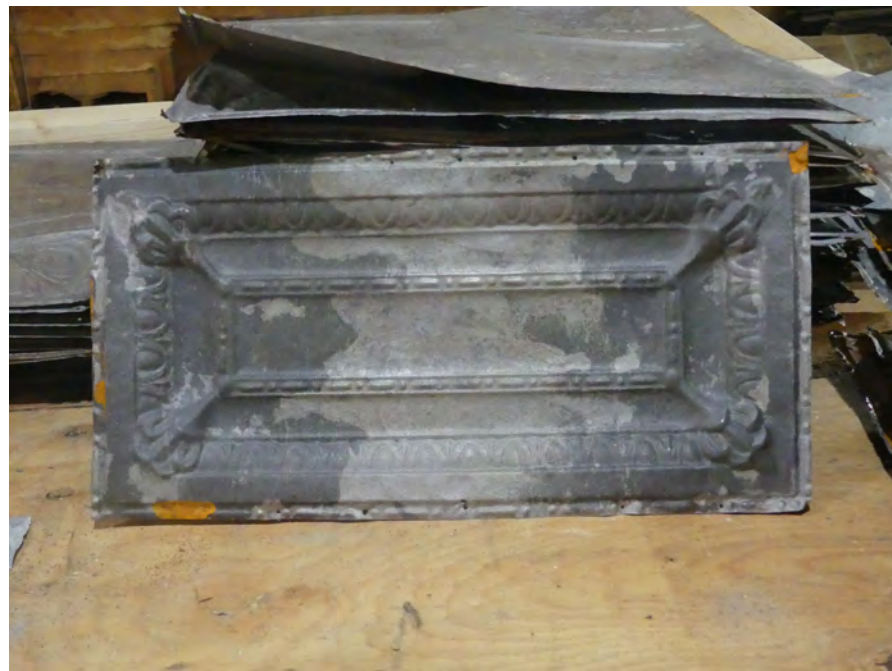
B. typical beam panel: 11 1/2 x 23 1/2 net size, 12 1/2 x 24 1/2 overall size total number of panels required: panels available in usable condition: 38 replacement panels required:
