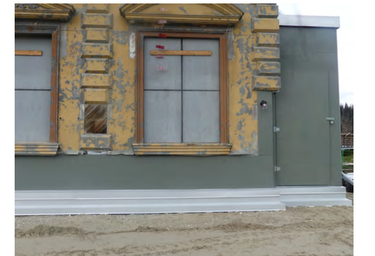
18. cornice, north east corner, some of the joint in the metal have opened, it is recommended that they be repaired in situ
