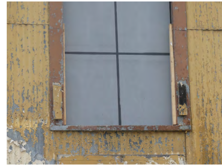
37. typical upper floor window frames, constructed from simple sheet metal forms
