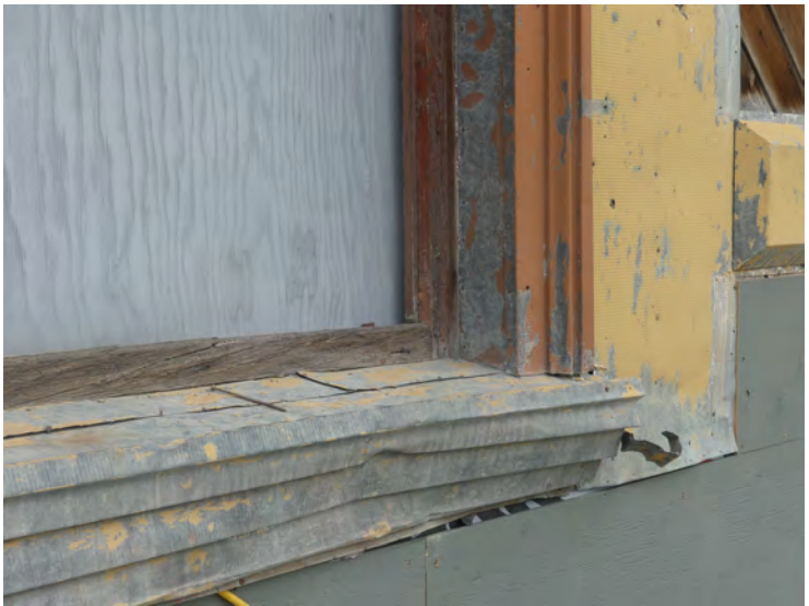
27. damaged sill, repair would likely require removal. Note the assembly with several pieces of overlapping metal. In some areas the sills fit around the siding, in others the siding runs beneath
