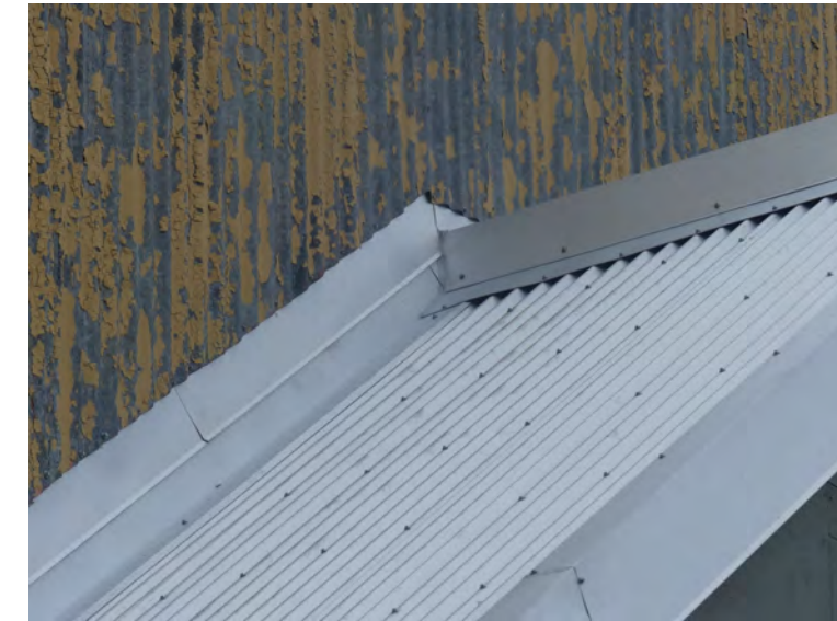
46. flashing detail
