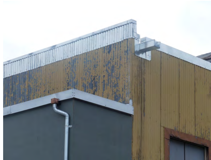
47. connection to the existing building, some flashing and cladding details should be modified to better reflect the original construction
