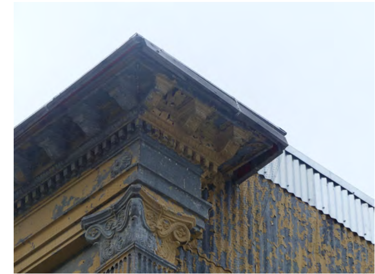
18. cornice, north east corner, some of the joint in the metal have opened, it is recommended that they be repaired in situ
