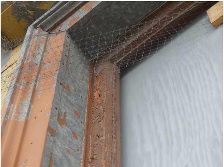
31. metal window trim and frame, typical
