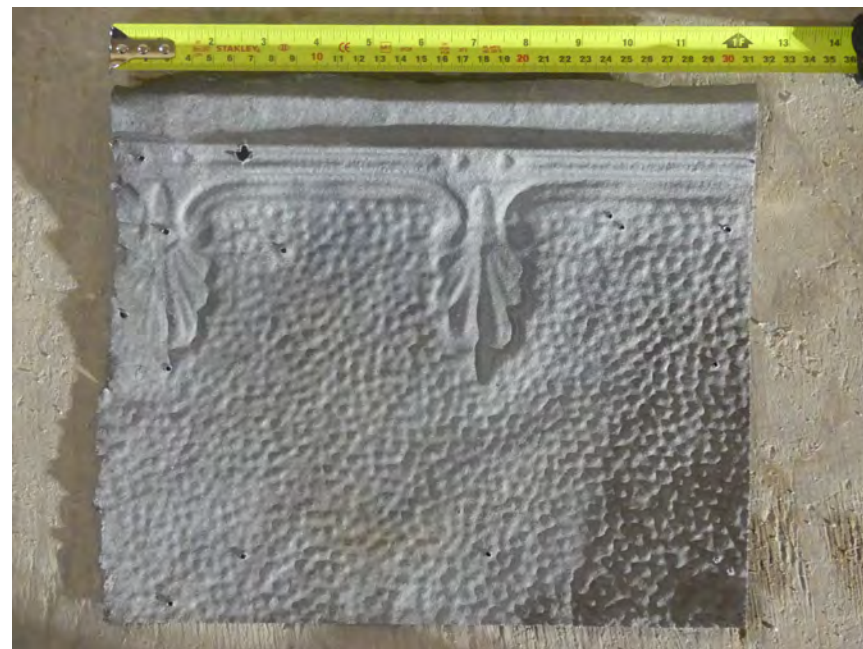
I. frieze: on wall: approx width 12" total lineal footage required: lengths available in usable condition: 96", 11 of: 88 ft 60", 2 of: 10 ft
