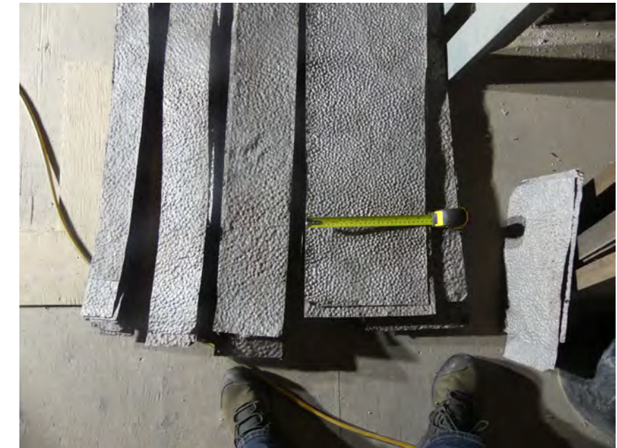
K: other horizontal filler pieces, variable widths and lengths to suit gaps, replace all
