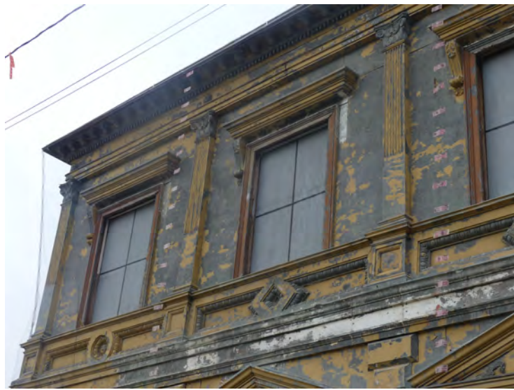
15. upper wall, generally intact, some quoins missing, The original paint color shows where the sign was located
