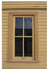
**Figure 4-30:** Exterior of typical main floor replica blind window on the south elevation. [PCA, 2018]
