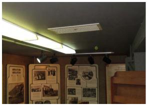
Figure 4-86: Exhaust grille at ceiling of ground floor
