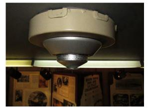
Figure 4-45: Heat Detector (Restorable) Ground Floor
