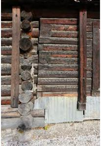
**Figure 4-21:** Detail of the building envelope on the south elevation depicting various construction styles, previous repairs and materials (at Area 3 and Area 4). [PCA, 2018]
