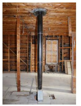
Figure 4-84: Exhaust duct through second floor up to roof
