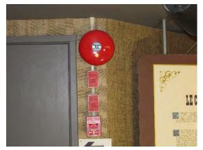
**Figure 4-44:** Signaling Device / Manual Station / End-of-Line Resistors
