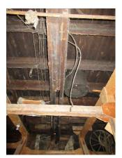
Figure 4-55: Loft Floor Assembly, Seen From the Ground Floor
