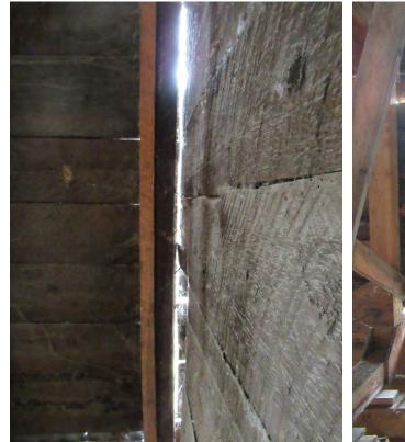
**Figure 4-8:** No connection between the exterior wall structures was observed between the first and second structure.
