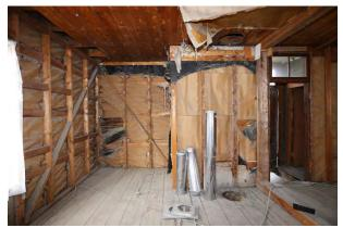
**Figure 4-41:** Second floor with evidence of water staining on walls and ceiling as well as remnants of former heating system. [PCA, 2018]
