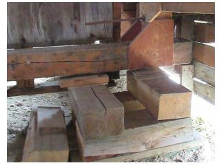
**Figure 4-6:** Concentration of shims along the south elevation of the interior frame.
