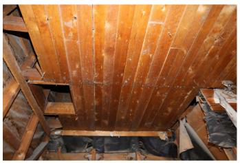
Figure 4-50: Second Floor Ceiling Assembly
