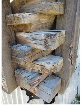
Figure 4-11: Deteriorated log ends on the fourth structure.
