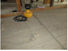
Figure 4-93: Electrical BX and EMT conduits
