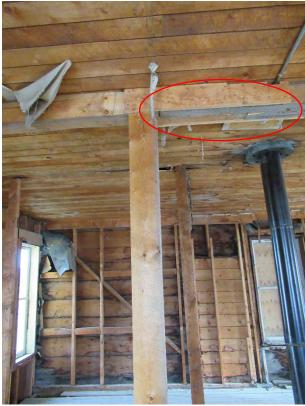
**Figure 4-12:** Lap joint (highlighted in red) observed offset from column. [PCA, 2018]
