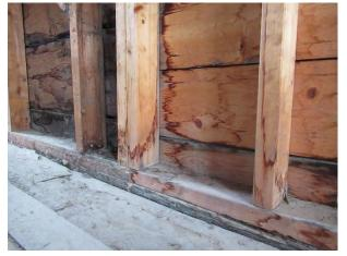
Figure 4-9: Moisture staining along the base of studs. [PCA, 2018]
