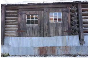
**Figure 4-28:** Wood double doors complete with windows found at the east end of the north elevation on Area 4. [PCA, 2018]
