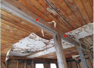
Figure 4-10: Large check on the underside of upper beam. [PCA, 2018]
