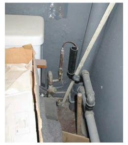
**Figure 4-79:** Toilet, sanitary drainage & water supply pipes. [PCA, 2018]
