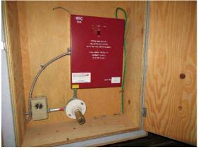
Figure 4-48: Fire Alarm Signal Transmitter / Control Unit (ESC 8240)
