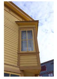
**Figure 4-20:** Side of the bay window where trim and siding have separated or cracked. [PCA, 2018]
