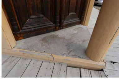
Figure 4-19: Condition of the threshold at the front entrance. [PCA, 2018]
