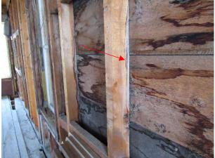
**Figure 4-8:** Moisture staining along edge of studs abutting exterior sheathing. [PCA, 2018]
