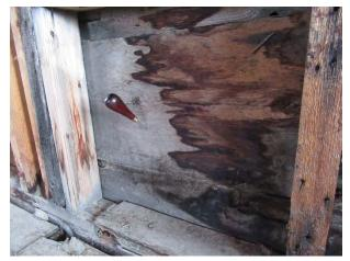
Figure 4-7: Moisture staining on exterior sheathing. [PCA, 2018]
