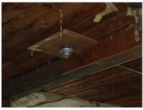
Figure 4-46: Heat Detector (Restorable) 2nd Floor
