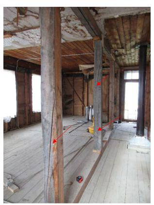
Figure 4-11: Spiral checking observed on columns. [PCA, 2018]
