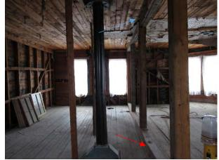
Figure 4-6: Central support spanning the length of the floor. Note the presence of two beams: upper beam (blue arrow), and lower beam (red arrow). [PCA, 2018]
