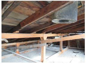
Figure 4-54: Loft Floor Assembly, Seen From the Loft
