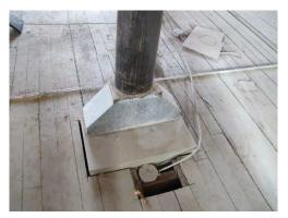
**Figure 4-58:** Floor Assembly Penetrations and Openings into Ground Floor Ceiling.
