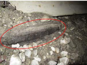
**Figure 4-4:** Shimming installed to stabilize rotation of supported beam. [PCA, 2018]
