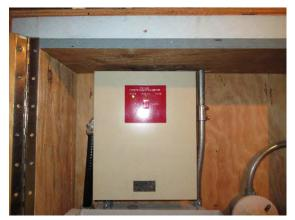
Figure 4-47: Fire Alarm Signal Transmitter (ESC 8240)
