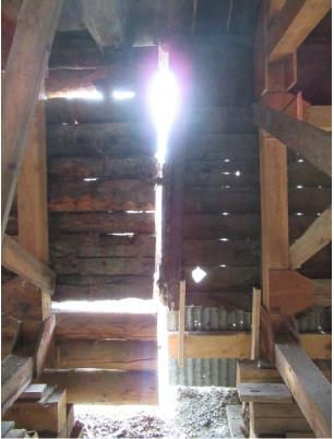
**Figure 4-9:** No connection between the exterior wall structures was observed between the third and fourth structure.
