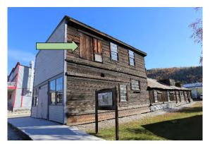
**Figure 4-67:** Fire Department Access to 2<sup>nd</sup> floor (Loft Area)
