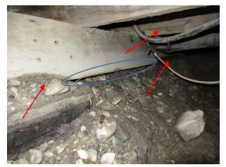
**Figure 4-3:** Localized moisture staining on the beams and joists (highlighted in red). Note that the staining on areas in contact with the soil is darker. Also note a portion of the beam without full bearing on the soil (highlighted in blue). [PCA, 2018]
