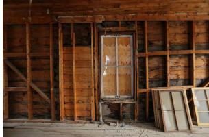
**Figure 4-42:** 2<sup>nd</sup> floor north wall illustrating boarded window with bird nest and exterior alterations. A set of unidentified windows was found. [PCA, 2018]
