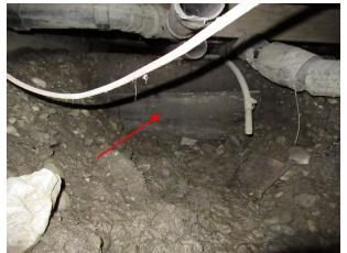
**Figure 4-2:** Localized excavated area by the access hatch. Vertical plywood retaining wall highlighted in red. [PCA, 2018]
