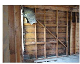
Figure 4-5: Typical stud wall construction on the second level. [PCA, 2018]
