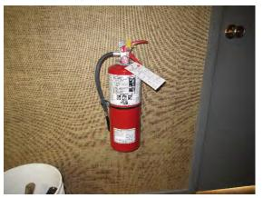
Figure 4-48: Portable Fire Extinguisher (Dry Chemical ABC)
