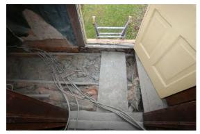
Figure 4-94: BX wiring on floor
