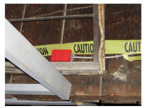
Figure 4-50: Initiating Circuit End-of-Line Resistor
