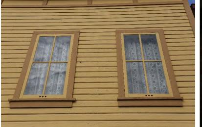
**Figure 4-27:** Exterior of typical second floor windows (storms) on the south elevation. [PCA, 2018]
