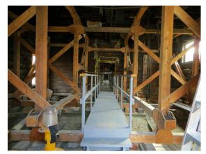
Figure 4-56: Structural elements supporting the building and 2<sup>nd</sup> floor, Loft floor assembly
