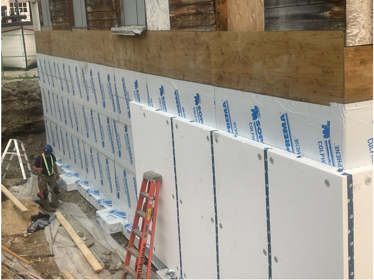
Figure 6: Installation of insulation
