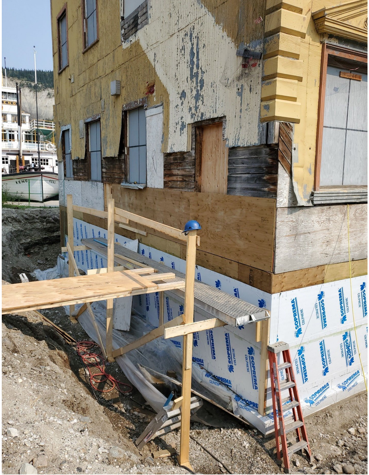
Figure 5: Installation of waterproof membrane
