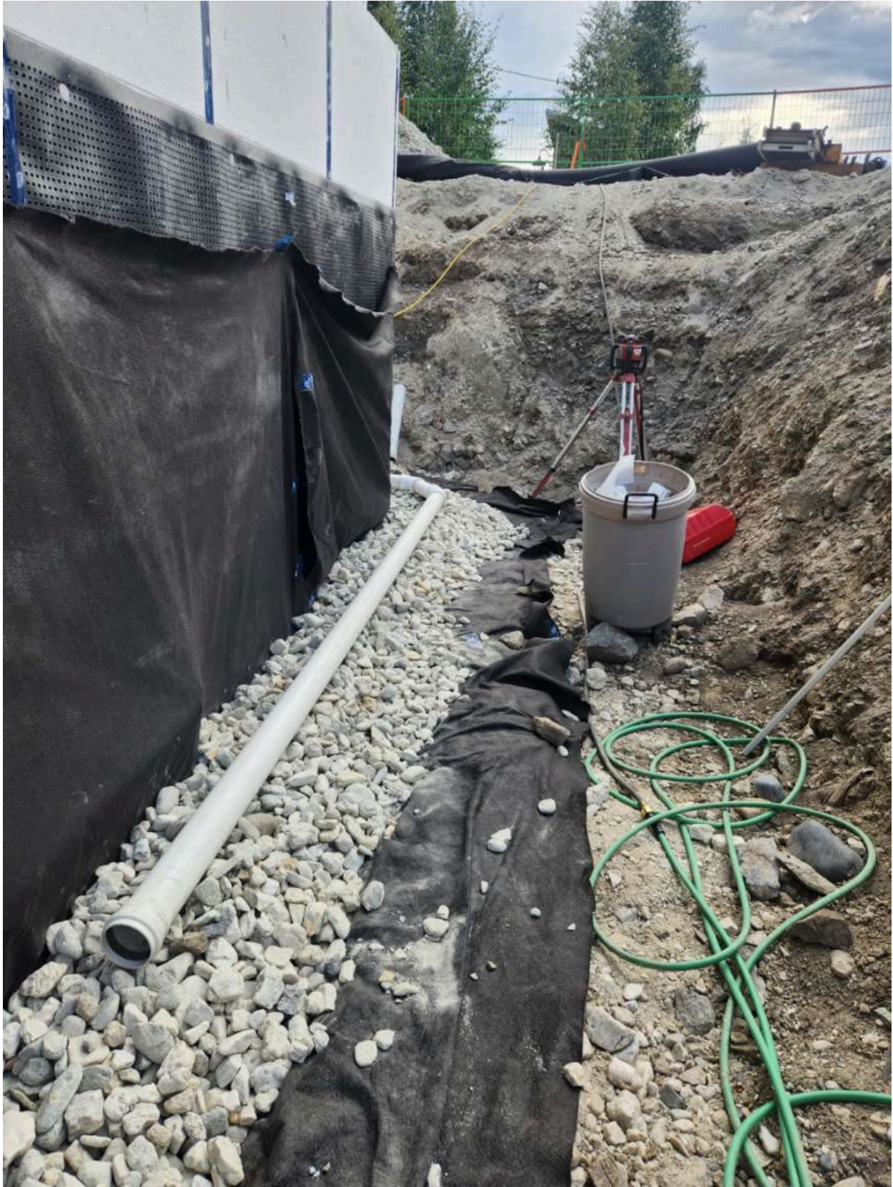
Figure 7: Installation of dimpled membrane and foundation drain
