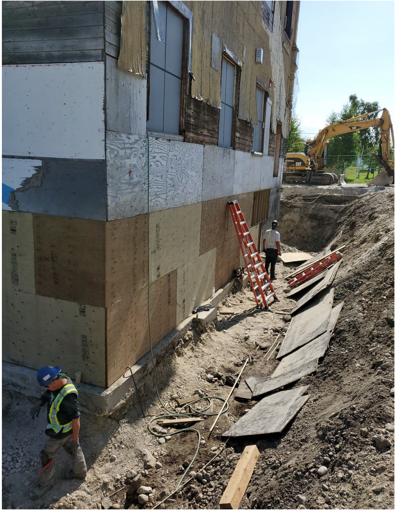
Figure 3: Plywood replacement
