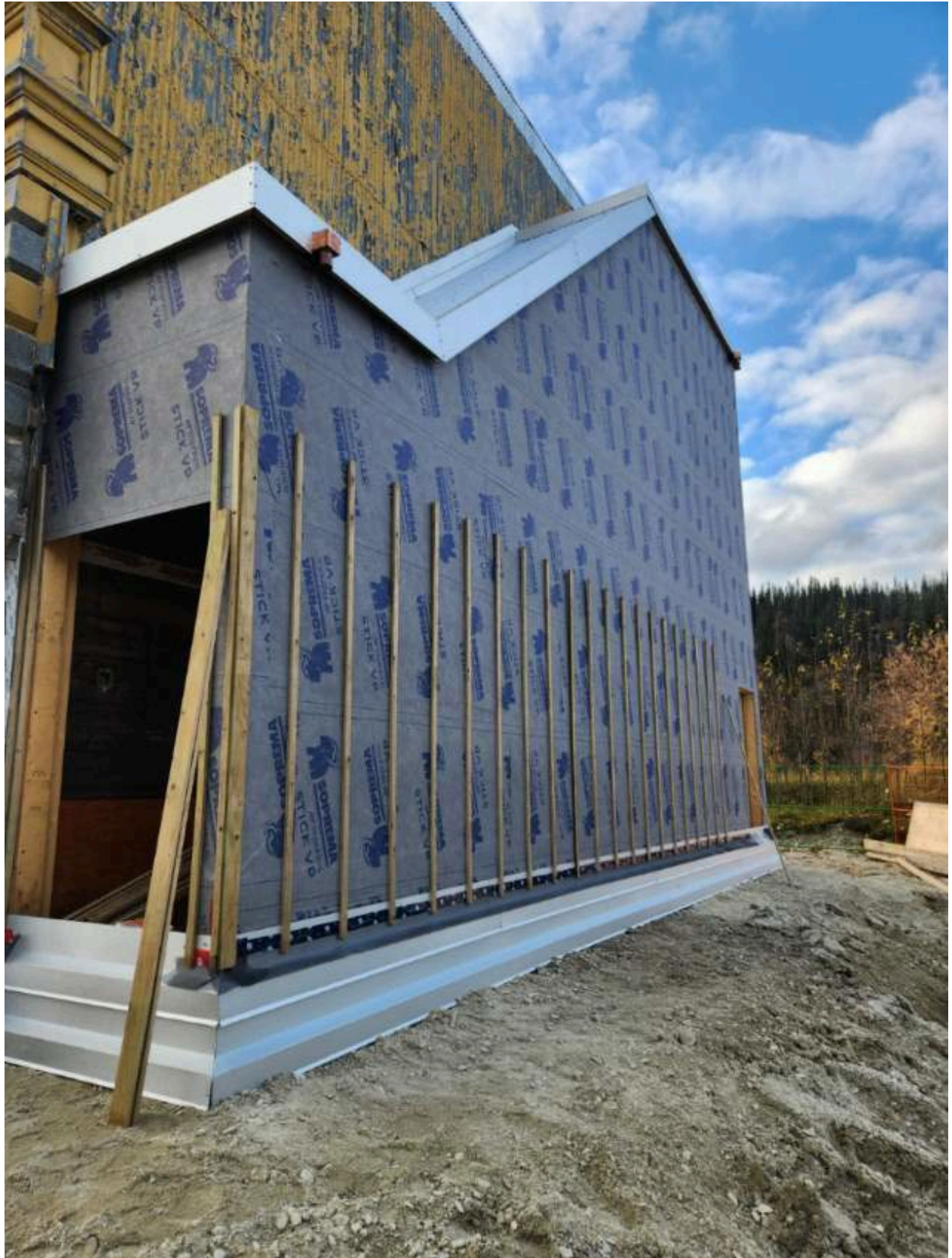
Figure 15: Extension roof completion
