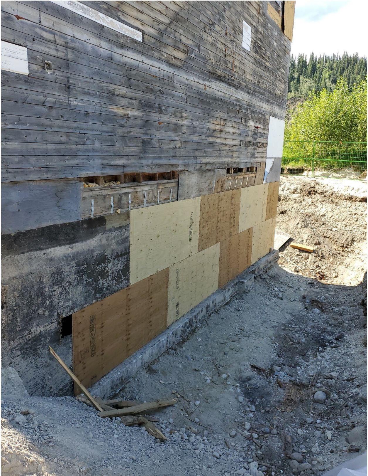
Figure 2: Plywood replacement
