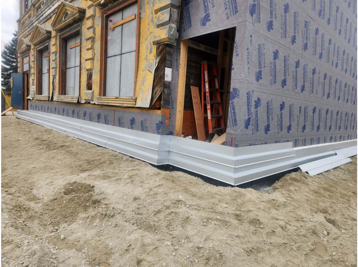
Figure 14: Backfill and skirting
