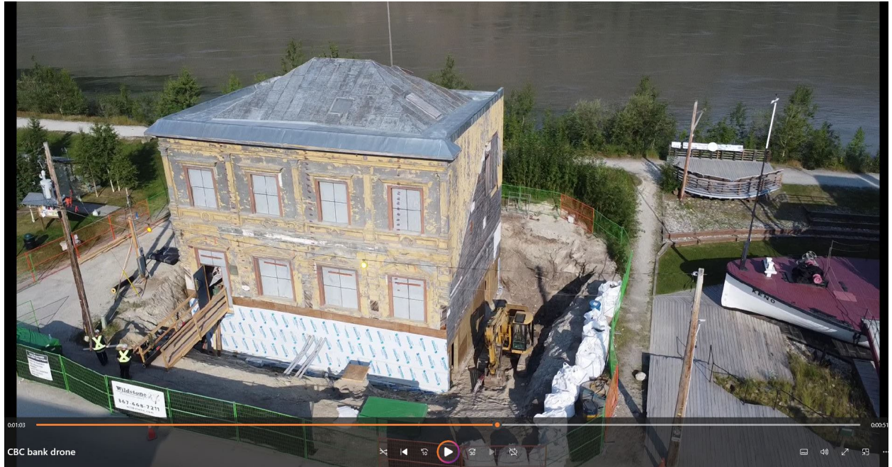
Figure 18: Drone footage during construction
