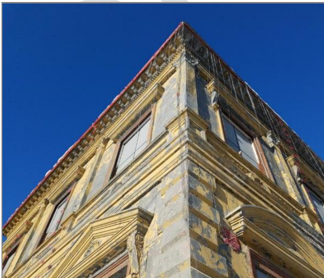
Figure 4.7 Pressed metal elements at southeast corner were generally sound.
