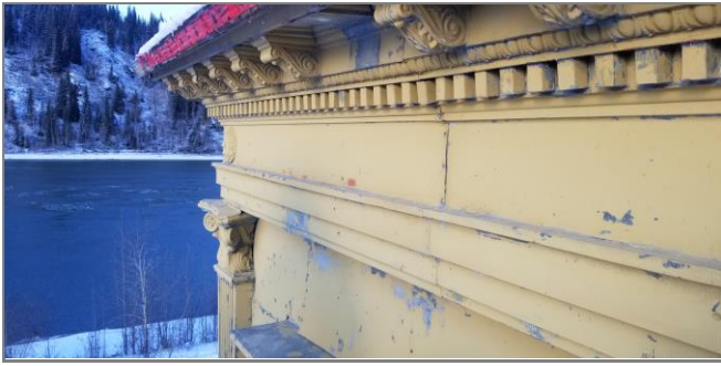
Figure 4.3 Stamped metal architectural elements at the roof line of the building.
