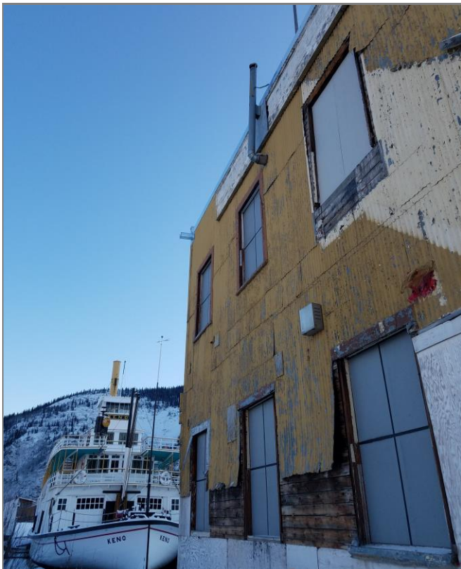
Figure 4.17 Window openings at the west elevation.
