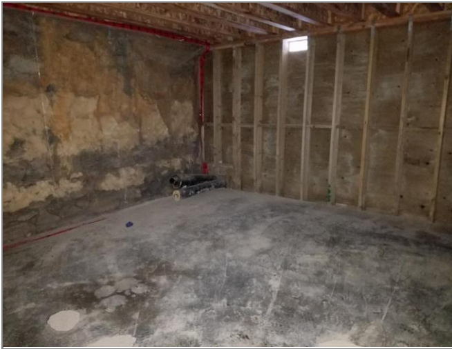
Figure 4.23 Basement looking northwest (vault visible left, sewer water hookup visible centre)
