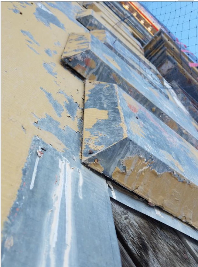
Figure 4.5 Quoin at field of wall.
