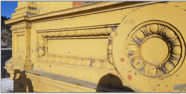
Figure 4.4 Stamped metal architectural elements between the first and second floors.
