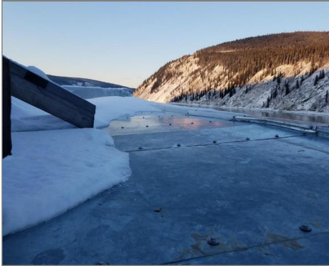
Figure 4.19 Metal roof assembly with gasketed roofing screws installed at seams.
