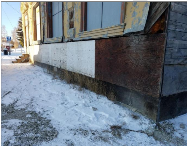
Figure 4.9 East elevation at grade transition to plywood sheathing.
