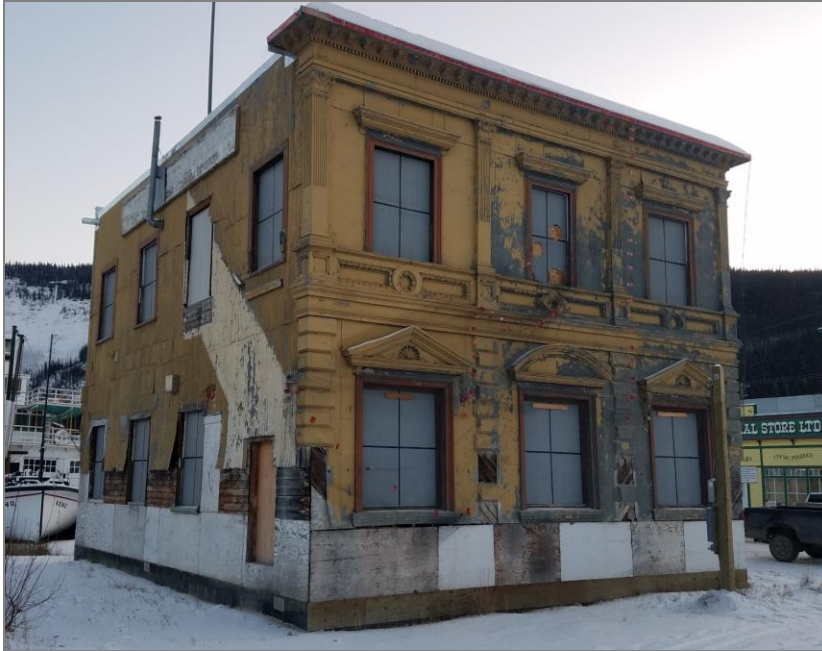
Figure 4.1 Southwest corner of the building.
