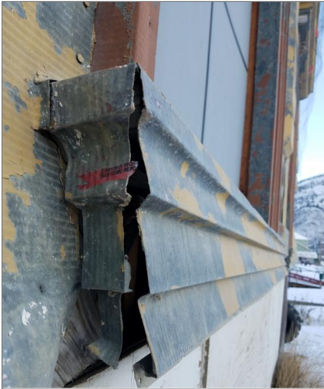
Figure 4.8 Typical window trim with open joints.
