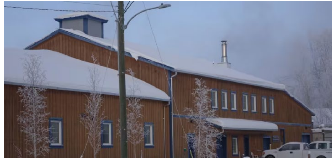
City of Dawson Wastewater Treatment Plant (Photo: CBC)
