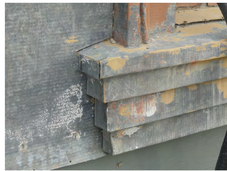
29. detail of sill and siding
