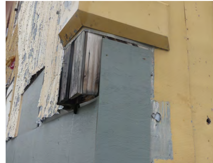
14. corner from south, showing backing and temporary plywood wall protection
