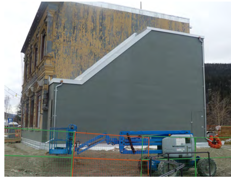
45. general view of reconstructed stair
