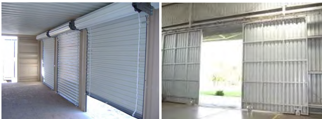
Figure 22: Garage Style Roll Up Door and Sliding Door
