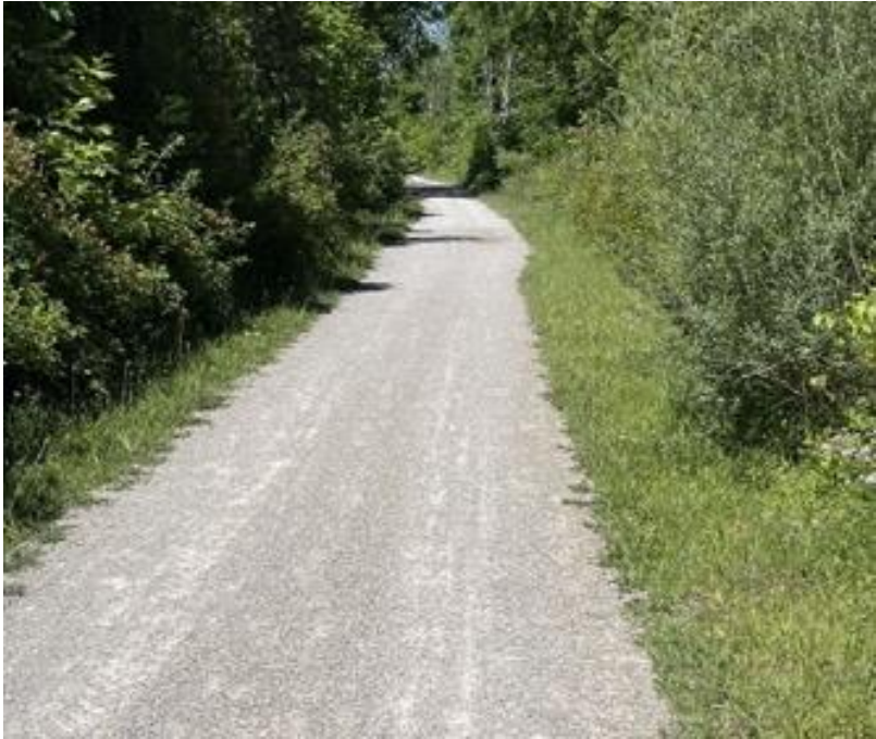
FIGURE 11: PROPOSED SURFACE MATERIAL FOR TRAIL CONSTRUCTION: COMPACT CRUSH
