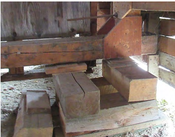
Figure 4-6: Concentration of shims along the south elevation of the interior frame.
