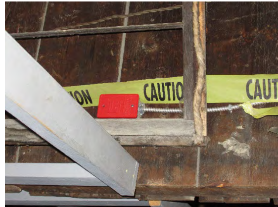
Figure 4-50: Initiating Circuit End-of-Line Resistor
