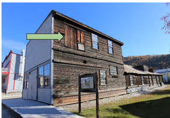
Figure 4-67: Fire Department Access to 2 nd floor (Loft Area)
