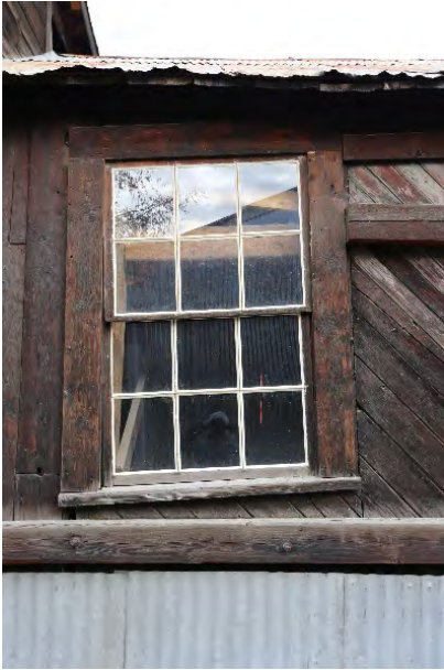
Figure 4-32: A typical but slightly skewed double hung window on south elevation of Area 2. [PCA, 2018]
