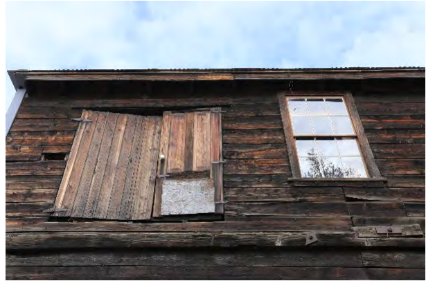
Figure 4-27: On the south elevation of Area 1 are remnants of the building's features from a time when Billy Biggs' had a full second floor. [PCA, 2018]
