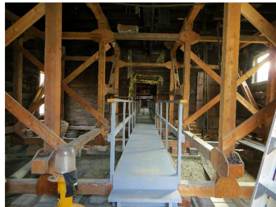
Figure 4-56: Structural elements supporting the building and 2 nd floor, Loft floor assembly
