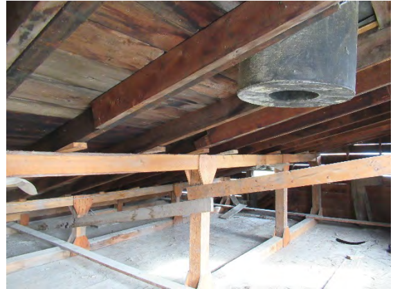
Figure 4-54: Loft Floor Assembly, Seen From the Loft
