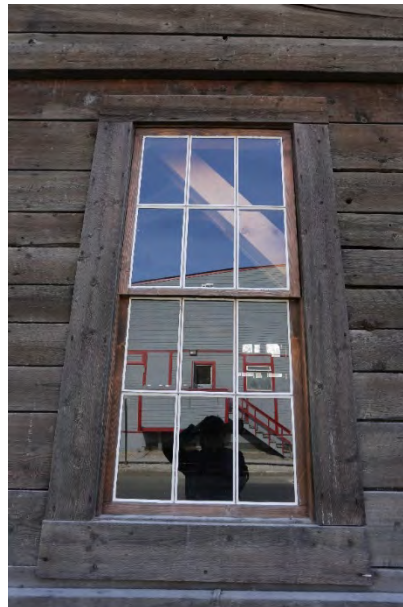
Figure 4-35: A double hung window found on the north elevation of Area 1. [PCA, 2018]
