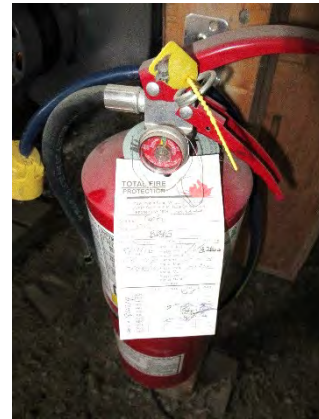
Figure 4-52: Portable Fire Extinguisher (Dry Chemical ABC)
