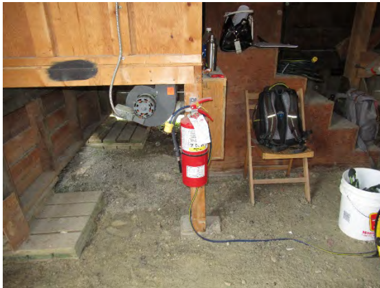
Figure 4-51: Portable Fire Extinguisher (Dry Chemical ABC)
