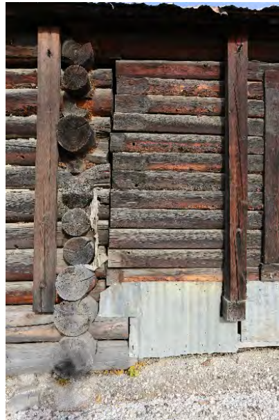
Figure 4-21: Detail of the building envelope on the south elevation depicting various construction styles, previous repairs and materials (at Area 3 and Area 4). [PCA, 2018]
