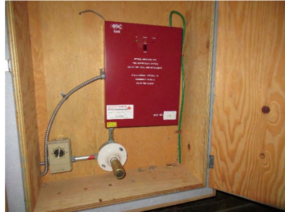
Figure 4-48: Fire Alarm Signal Transmitter / Control Unit (ESC 8240)
