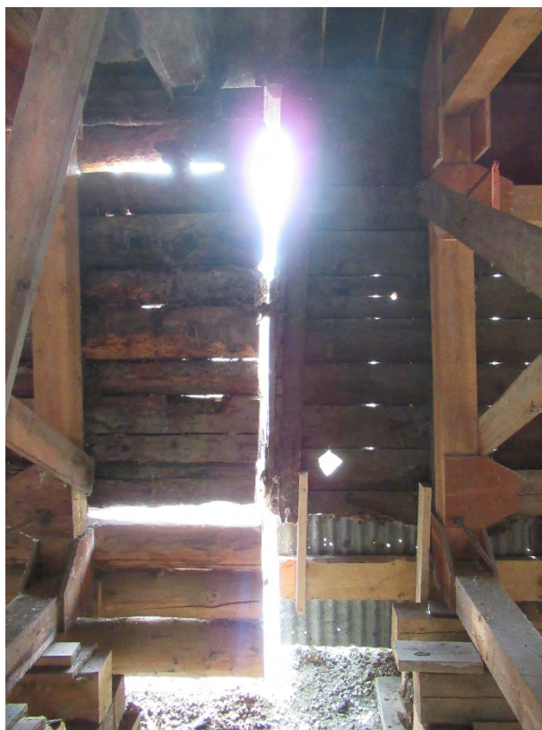
Figure 4-9: No connection between the exterior wall structures was observed between the third and fourth structure.
