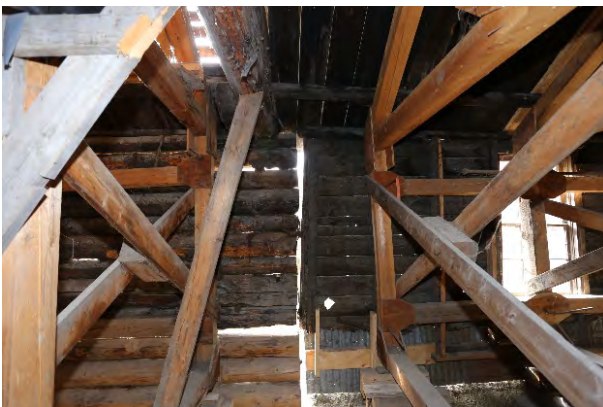
Figure 4-46: Interior view looking south of the junction between Areas 2 and 3. Previous log repairs are seen in the lower left of the photo. [PCA, 2018]
