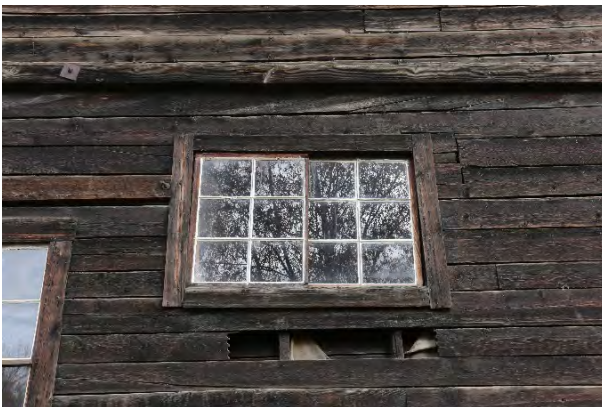
Figure 4-34: This double hung window found on the south elevation of Area 1 has been installed on its side. [PCA, 2018]
