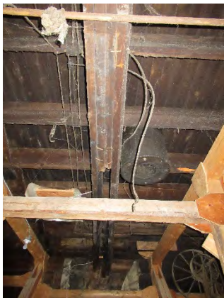
Figure 4-55: Loft Floor Assembly, Seen From the Ground Floor
