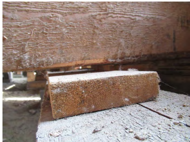
Figure 4-7: Shimming along the south and north elevations was observed to be loose. Note the gap between the shims and the underside of the interior frame.
