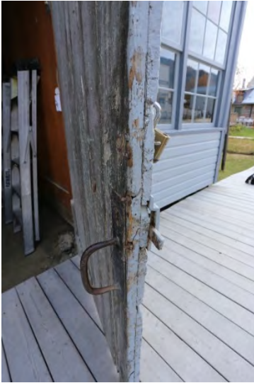
Figure 4-26: Construction and hardware of one of the wood front doors on west elevation Area 1. [PCA, 2018]
