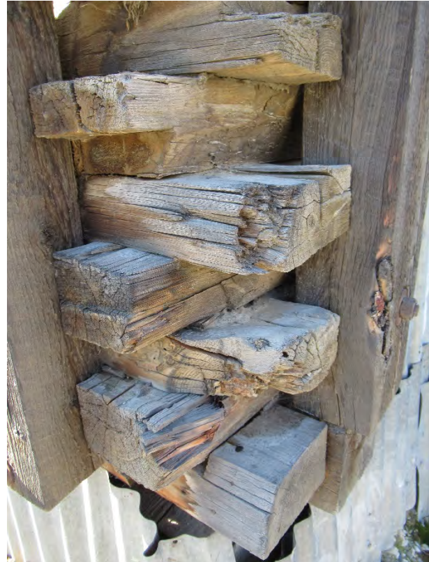
Figure 4-11: Deteriorated log ends on the fourth structure.
