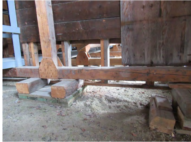
Figure 4-5: Minimal shimming along the center of the interior frame.
