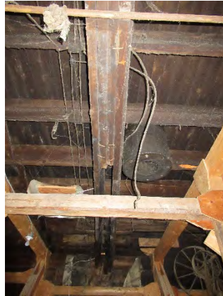
Figure 4-53: Loft Floor Assembly, Seen From the Ground Floor
