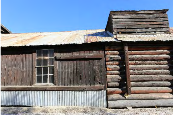
Figure 4-18: South elevation illustrating the different construction styles between Area 2 and Area 3. [PCA, 2018]
