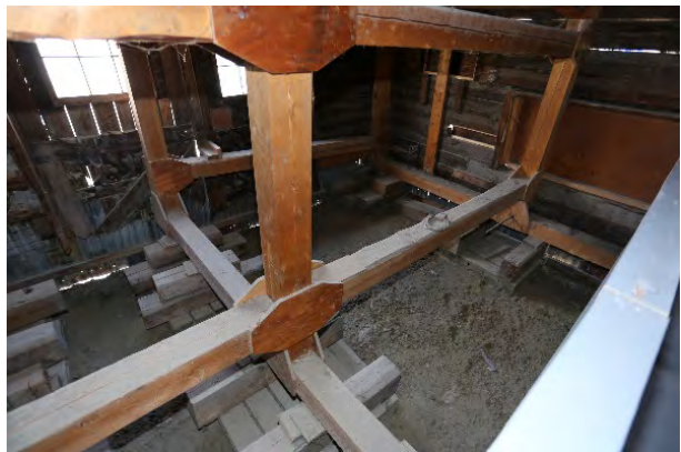
Figure 4-45: Typical flooring and bracing condition as found in Area 4. [PCA, 2018]
