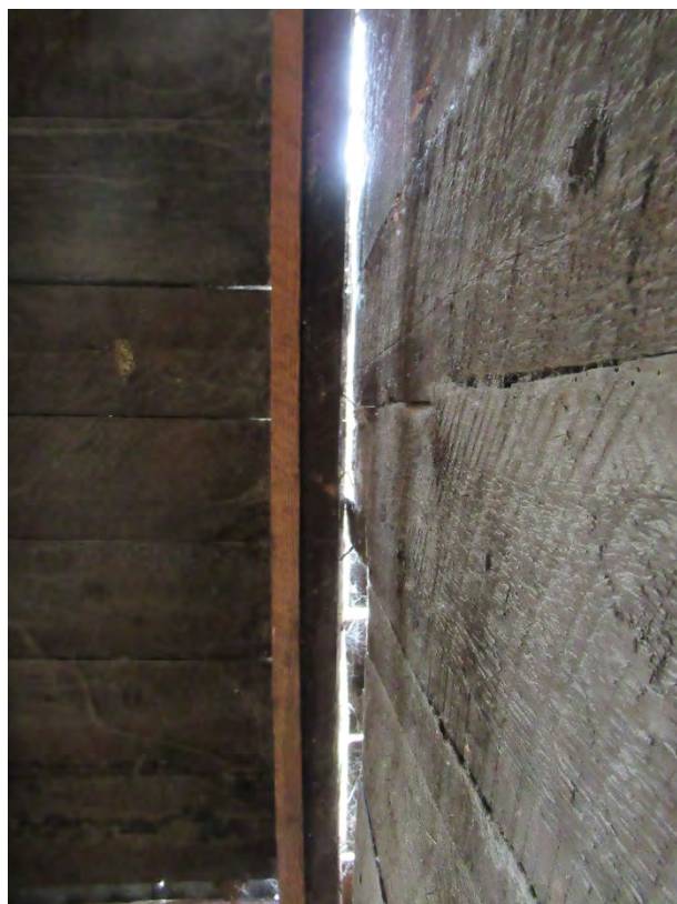
Figure 4-8: No connection between the exterior wall structures was observed between the first and second structure.
