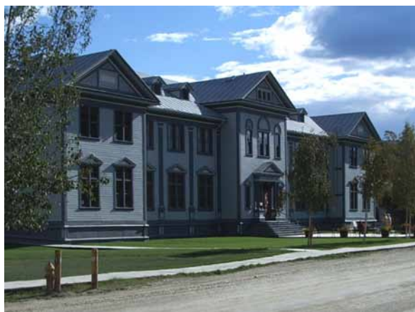
Old Territorial Administration Building, now the Dawson Museum, 2007, a Palladian-Georgian design that symbolized the authority of Government. (Photo: H. Kalman)
