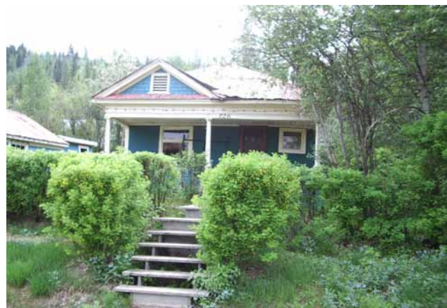
A house from the Gold Rush era, located on 8th Avenue near Harper Street, was demolished in October 2007. (Photo: H. Kalman)
