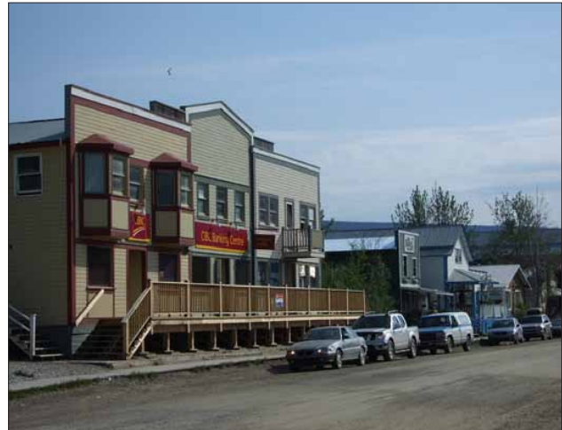
With its raised verandah and the ground floor set about 1 metre above grade, the CIBC is cut off from its neighbours and sits like an island with no easy interface with the boardwalk or street. Compare the lower siting of the old buildings to the right. (Photo: H. Kalman)
