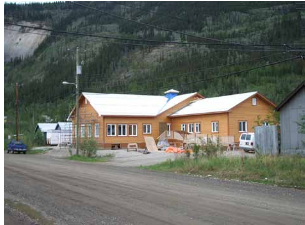
A day care centre built by the Tr'ondëk Hwëch'in on Second Avenue is one of a number of new buildings in the North End. (Photo: H. Kalman)
