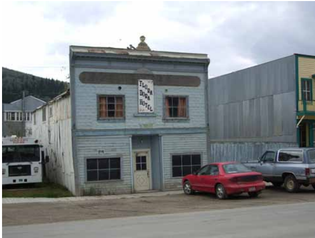
The Flora Dora Hotel is a survivor from the Gold Rush era. The structure remains empty. (H. Kalman)
