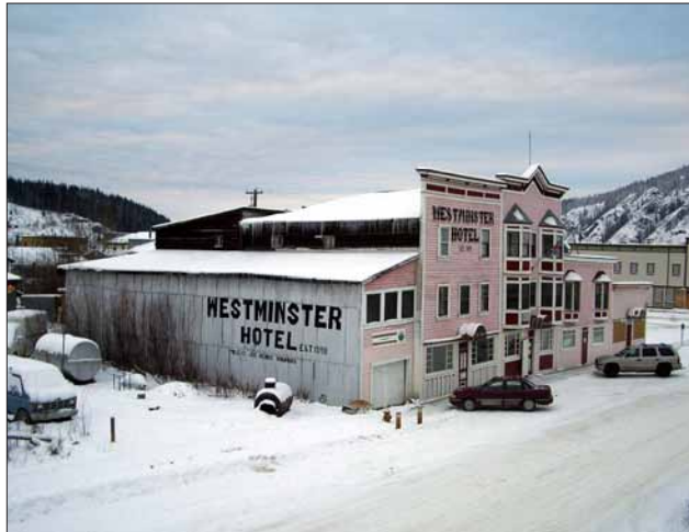
The historic Westminster Hotel on 3rd Avenue, built in stages from 1901 to the 1930s, is located on grade. This siting is pedestrian-friendly and retains heritage character, but risks damage from frost heaves and water.
