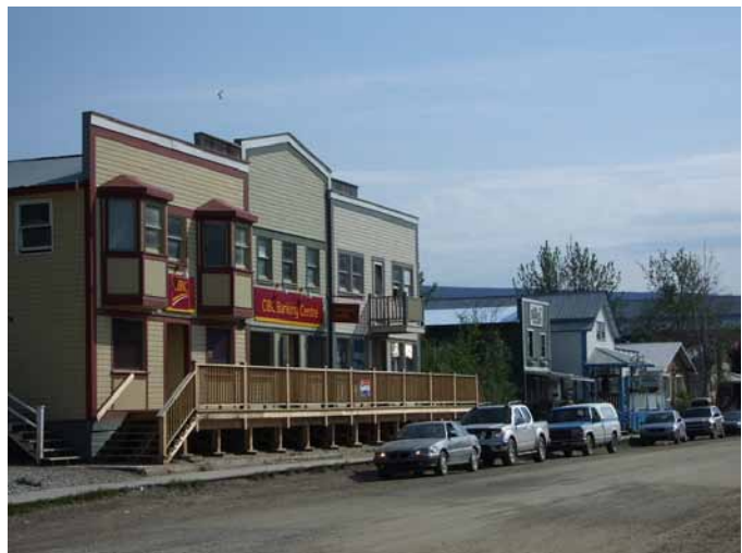
The CIBC on Second Avenue is a recent building with Gold Rush features. Its high ground floor and entrance walkway respect the flood plain but alter the streetscape. (Photo: H. Kalman)
