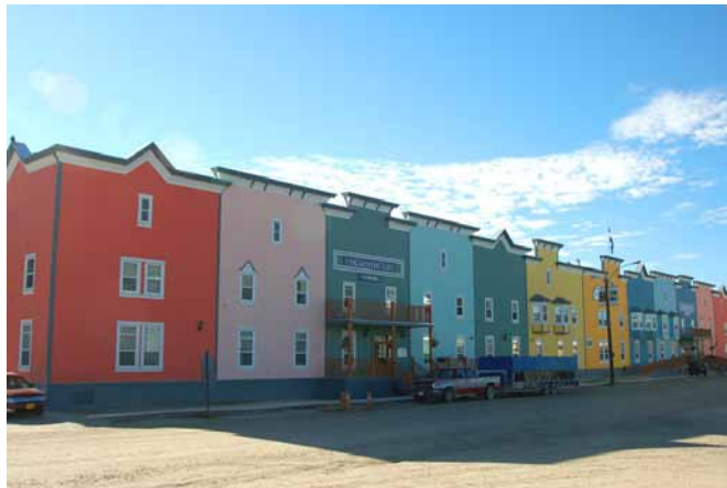
The Westmark Inn is a large building whose elevation has been treated as if it were a number of small, Gold Rush-era buildings; however, the uniform flatness of the wall and the design proportions lack any conviction. (Photo: H. Kalman)
