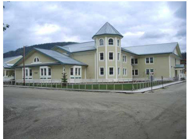
The Robert Service School / Dawson Public Library complex uses Gold Rush-era forms and details on a building whose scale is far greater than buildings from the historical period. (Photo: H. Kalman)
