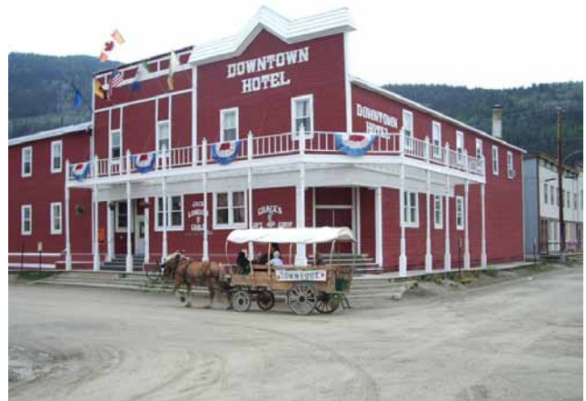
The Downtown Hotel was built in the early 1980s to accommodate increasing tourism. Its scale is larger than the Flora Dora and other Gold Rush buildings. (Photo: H. Kalman)
