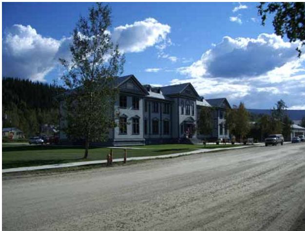
The Old Territorial Administration Building (now the Dawson Museum) is set in Minto Park, establishing the tone for government buildings and landscapes from the Gold Rush era. (Photo: H. Kalman)
