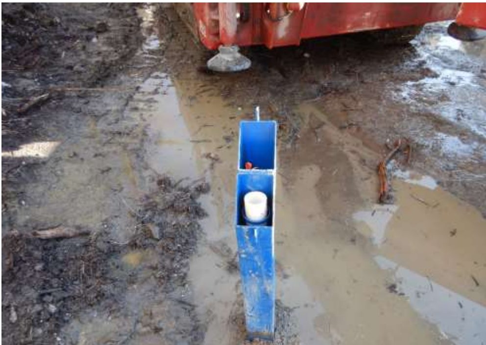
Photo 4: Completed MW20-03, 27 April 2020
