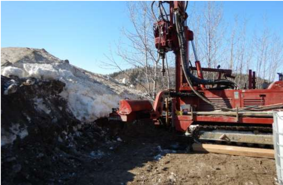
Photo 1: Drilling and installation of MW20-02, 25 April 2020
