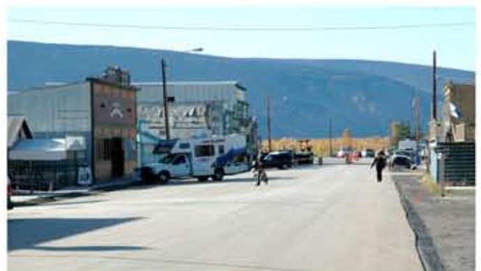
Front Street gets the top coat of clear pavement.
